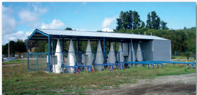
Oxygenenrichment at inlet to fishfarm
